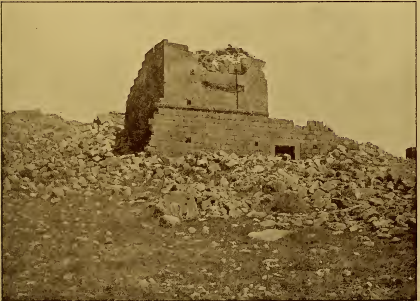
Part of a Monastery above Bin-Bir-Kilisse, showing short zones of brick used as ornament in a stone building.
